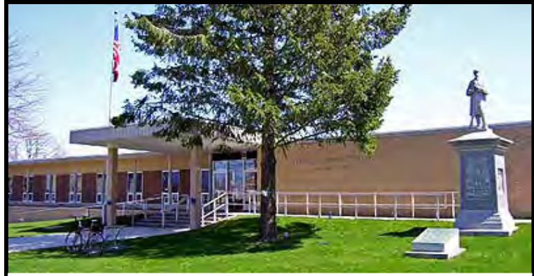
Oceana County Building
